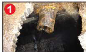
Before (Cast Iron Pipe)
