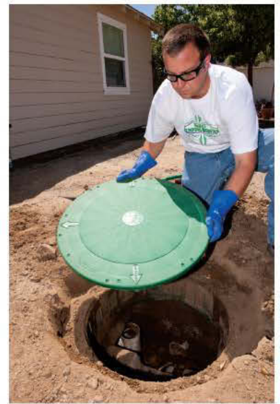
T.J. Miller installs a new Tuf-Tite riser for a residential customer. The Millers like when they can bring the tank lid to ground level to limit digging for system pumping and inspections.
