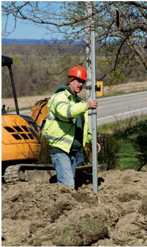
Sean O'Brien takes measurements while installing a new septic system drainfield.
