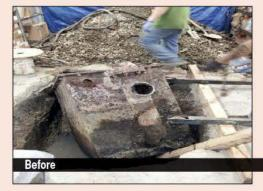
**Problem:** In May 2012, Norton Sewer Service was called to replace a corroded steel grease interceptor at an assisted living facility in Chicago. The 1,300-pound steel unit required a
