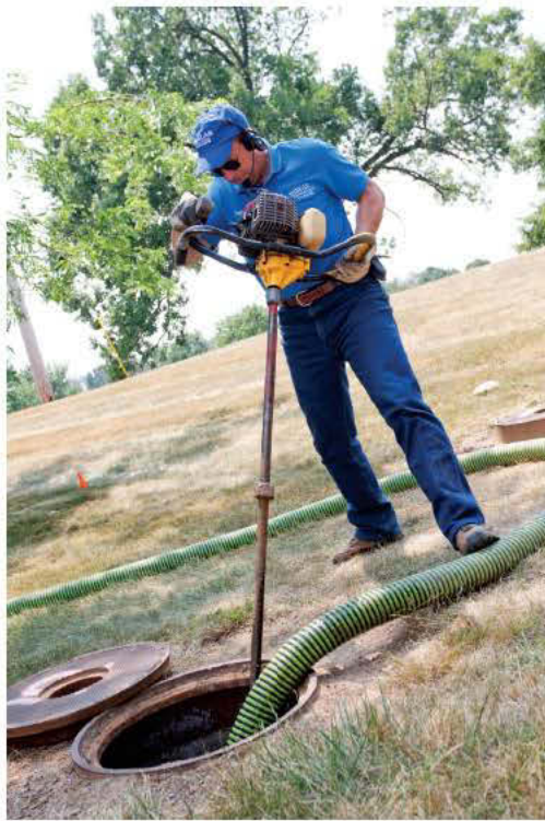
Duane Shelar uses a Crust Buster to liquefy a neglected tank with a heavy scum layer.
