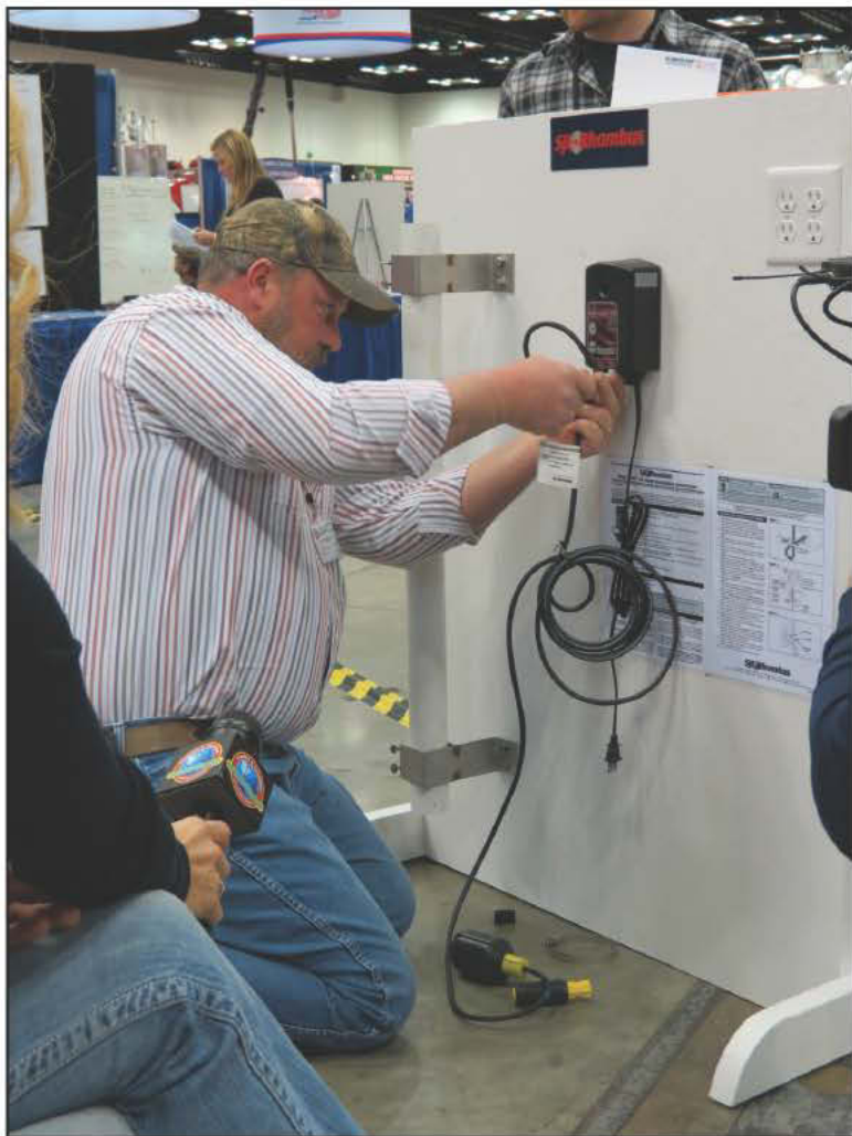
Many onsite system professionals competed to see who could install an SJE-Rhombus septic tank alarm the fastest. The winner received $100 from COLE Publishing and four passes to the 2013 Pumper & Cleaner Environmental Expo International.
