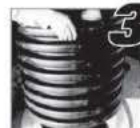
Place plastic maintenance pipe on ring.
