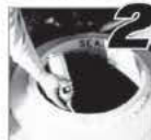
Place ring over opening and apply foam.
