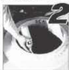
Place ring over opening and apply foam.
