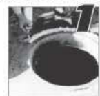
Apply foam sealant to tank.
