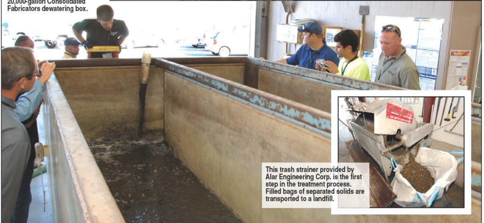
Owner Dean Trevaskis (upper left) watches a load of septage empty into a 20,000-gallon Consolidated Fabricators dewatering box.
