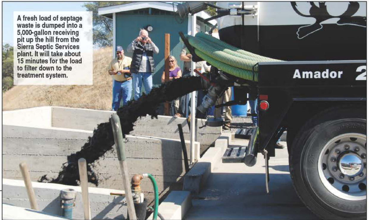
Owner Dean Trevaskis (upper left) watches a load of septage empty into a 20,000-gallon Consolidated Fabricators dewatering box.
