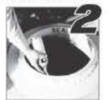
Place ring over opening and apply foam.
