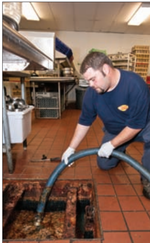
Jeremiah Burpo maneuvers a tight kitchen space with the Dyna-Lite (left), then gets to work emptying the grease trap.
