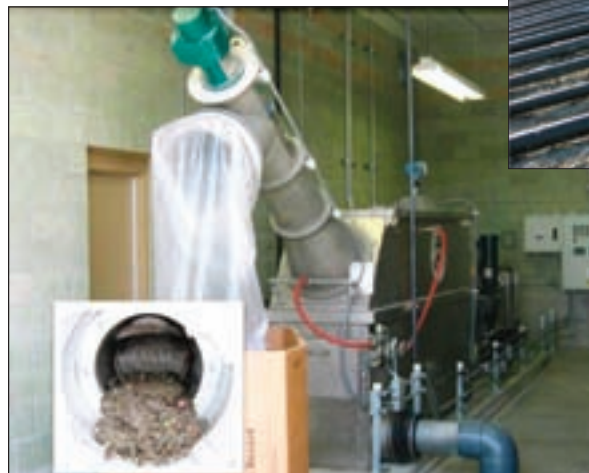
Left, a JWC Honey Monster removes solids from the septage. The bags of solids are buried in the landfill.
