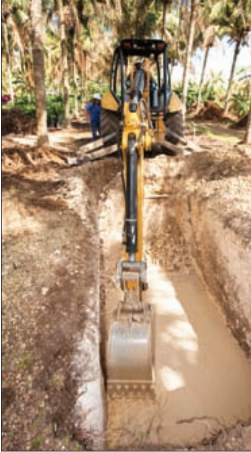
Anthony Sweat (above) uses a Caterpillar 430EW backhoe to place a new septic tank. At right, Nesenman checks the depth for proper septic tank placement.
