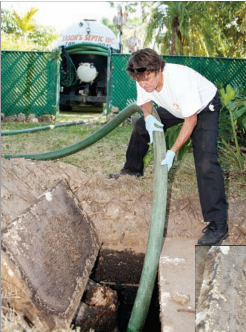
Tommy Edwards (above) pumps an aging septic tank before the crew can inspect the tank and make necessary repairs. At top right, Richard Aoci assembles a new outlet tee for the tank. Below right, the crew found that the original outlet had rotted away.
