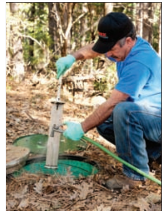
At left, Doug Urke unloads his Bobcat mini-excavator to excavate a septic tank lid for a service call. Above, Bob Zoellin cleans a septic filter.
