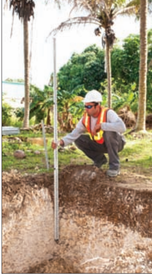
Anthony Sweat (above) uses a Caterpillar 430EW backhoe to place a new septic tank. At right, Nesenman checks the depth for proper septic tank placement.
