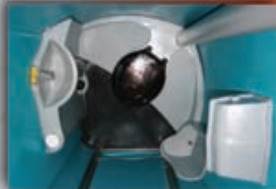
Interior View of TJ-III with sink
