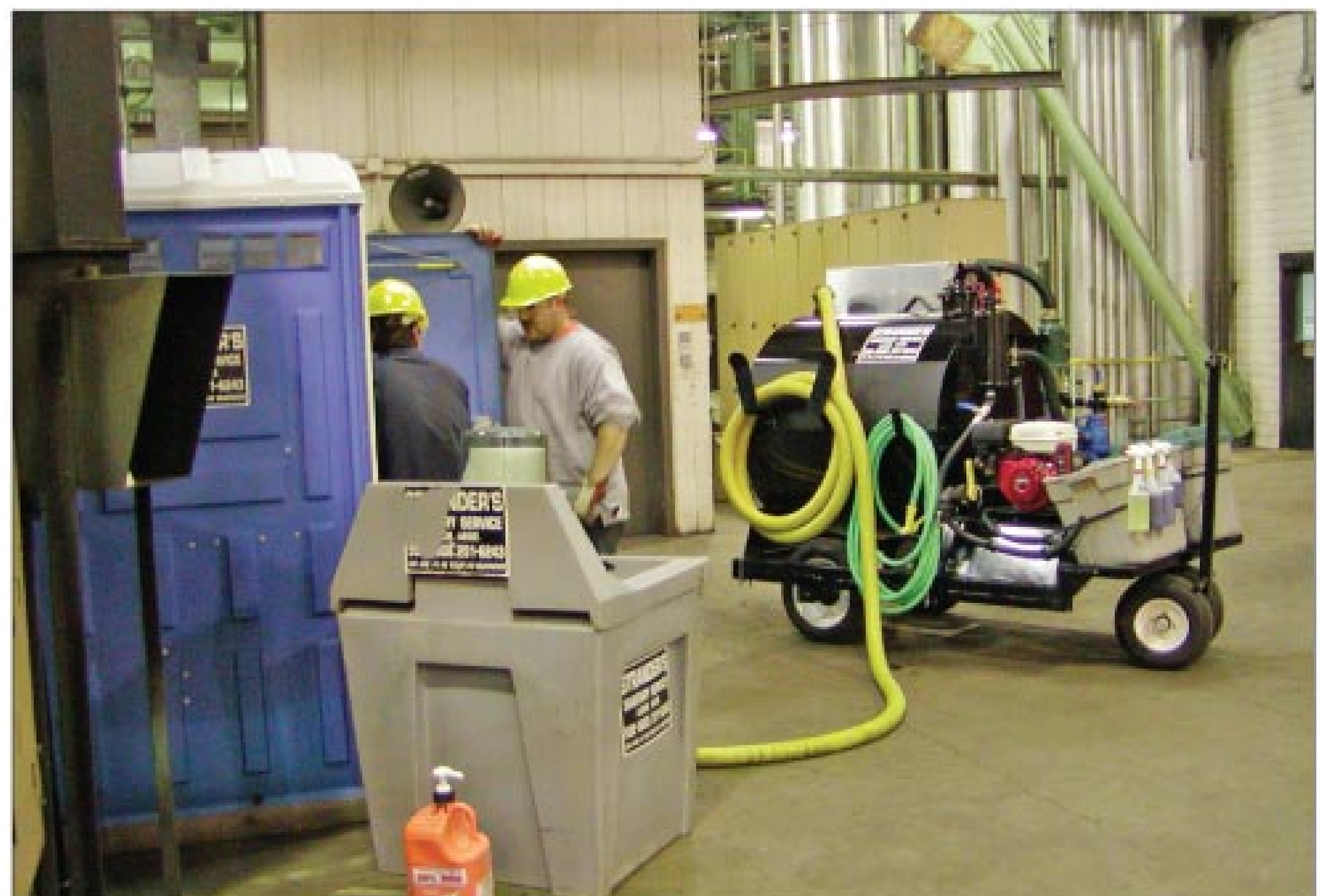
A service cart from Imperial Industries Inc. is used inside a plant where the only access to portable restrooms is by elevator. Burdine and Mike Gladem are the service techs.
