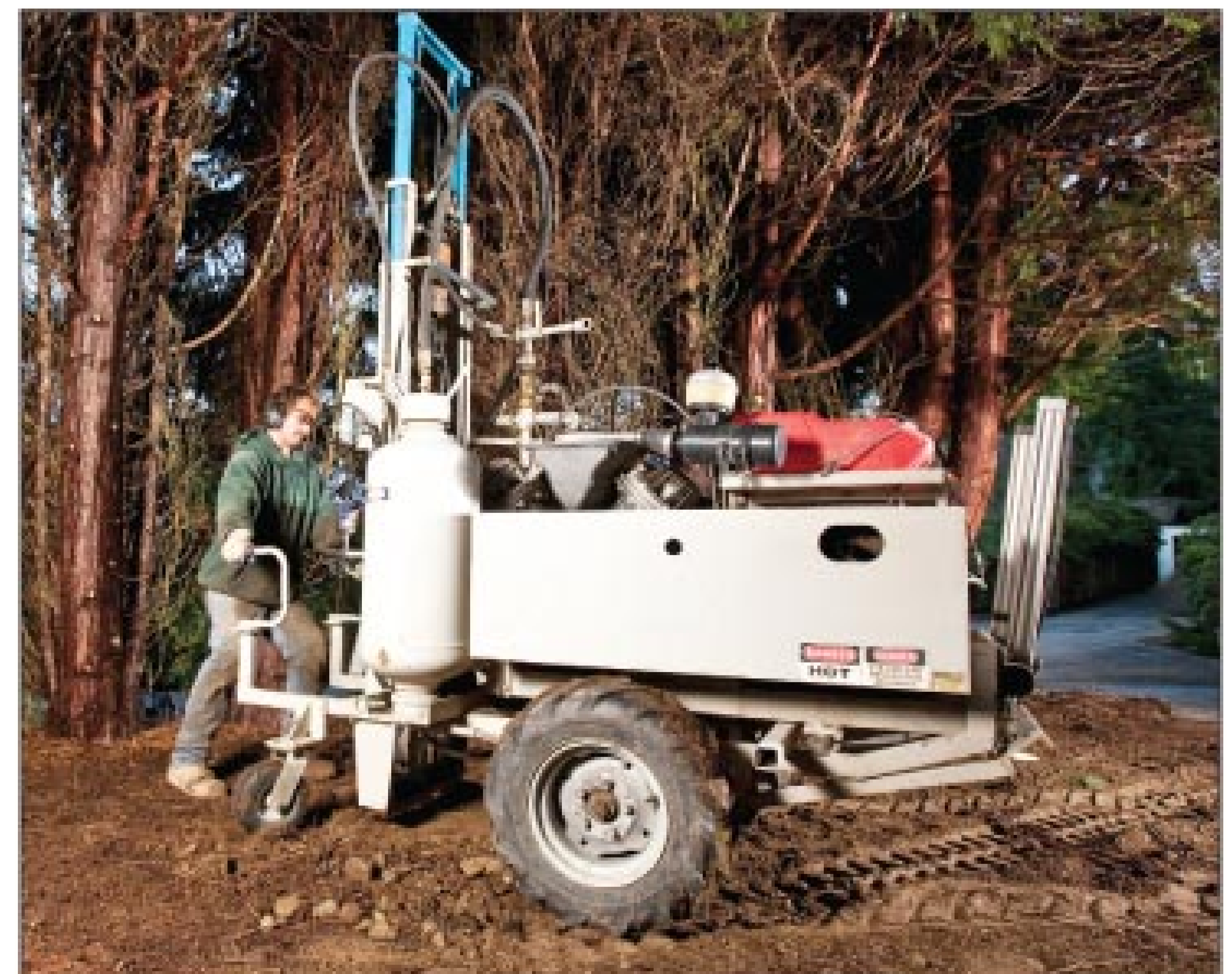
Above, Beaulieu uses a mini excavator to fill the trench surrounding a new inspection port and riser. At right, Simpson operates a Terralift machine to rejuvenate a drain field.
