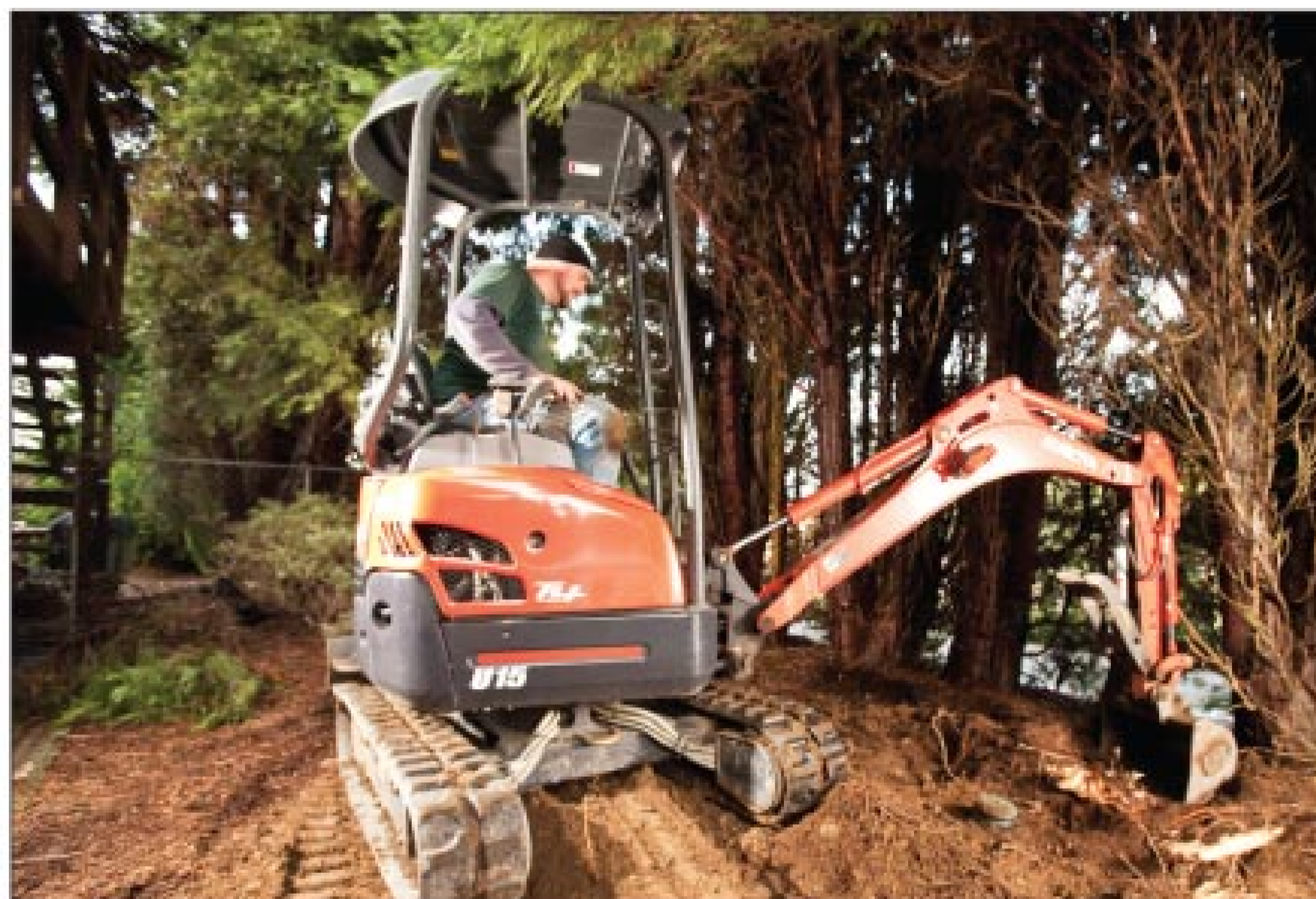
Above, Beaulieu uses a mini excavator to fill the trench surrounding a new inspection port and riser. At right, Simpson operates a Terralift machine to rejuvenate a drain field.
