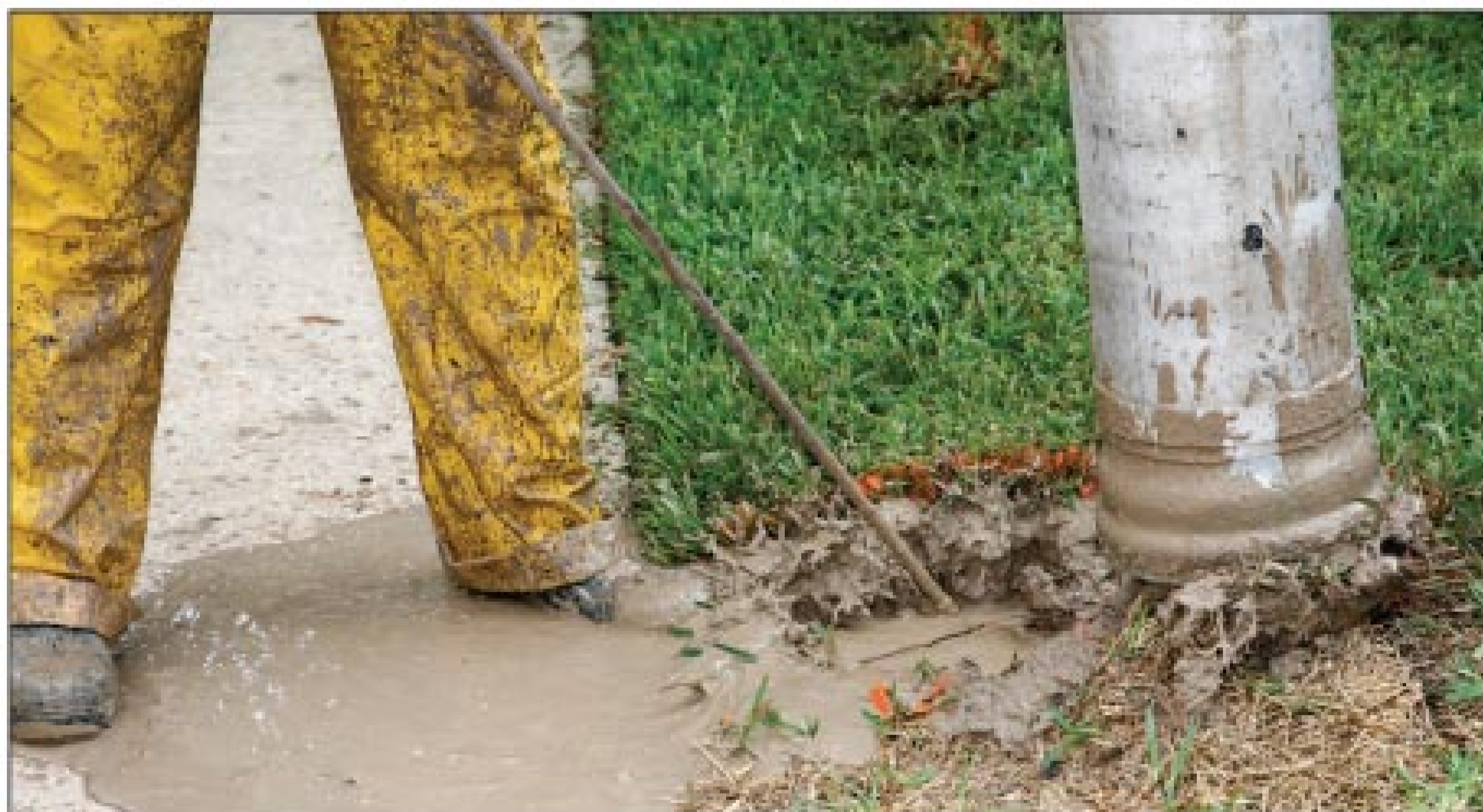
Water is jetted into each light pole hole, while mud is conveyed to the combination truck tank. At right, Rios and Pina monitor the hydroexcavation work.
