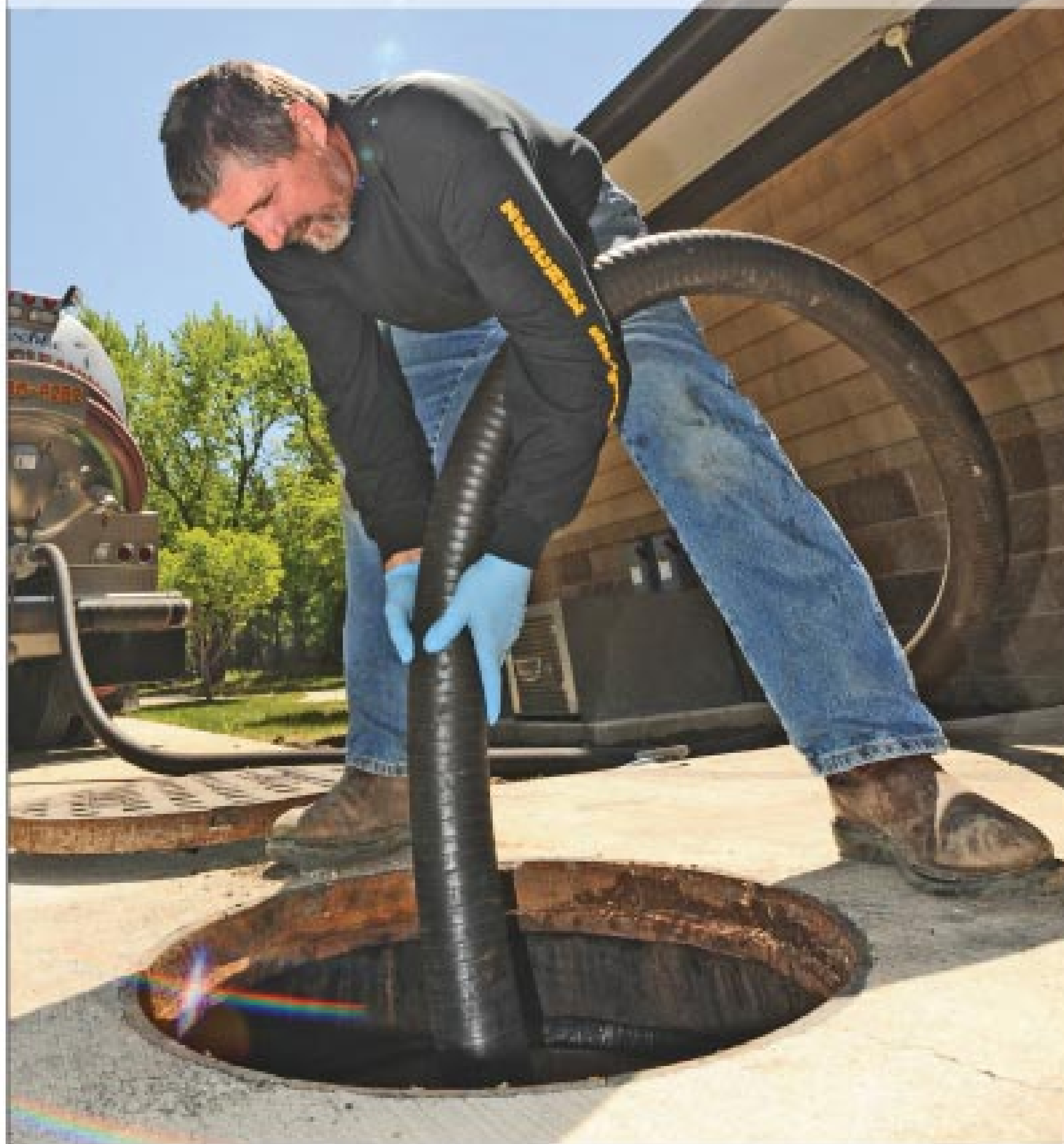
Cary Zeschke cleans a grease trap. Grease trap service has grown into about 30 percent of the company’s business in eight years.
