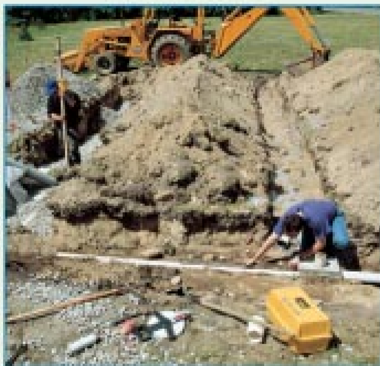
Typical Septic System Replacement Installation
