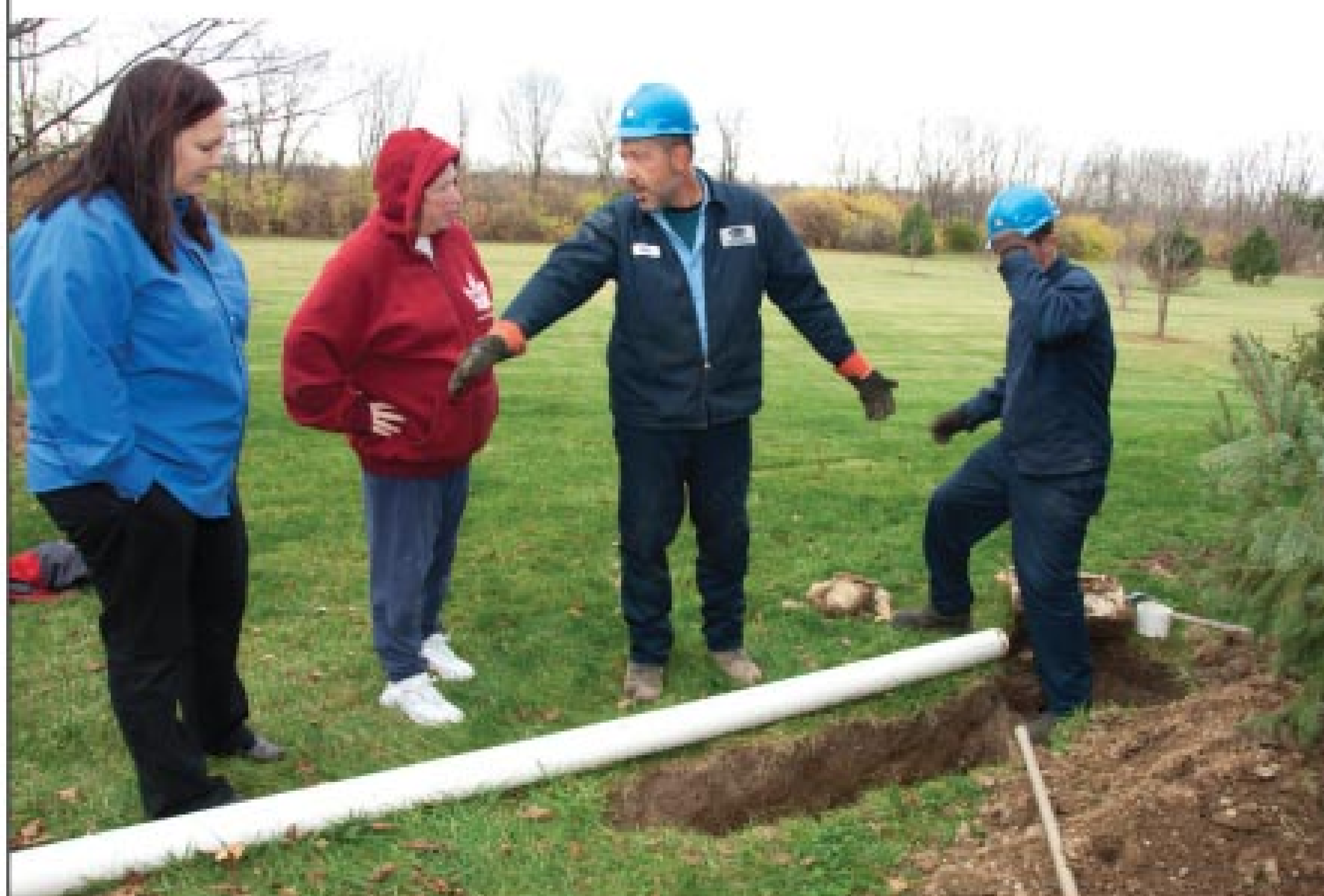
Marc Davis explains work on a septic system to a homeowner.
