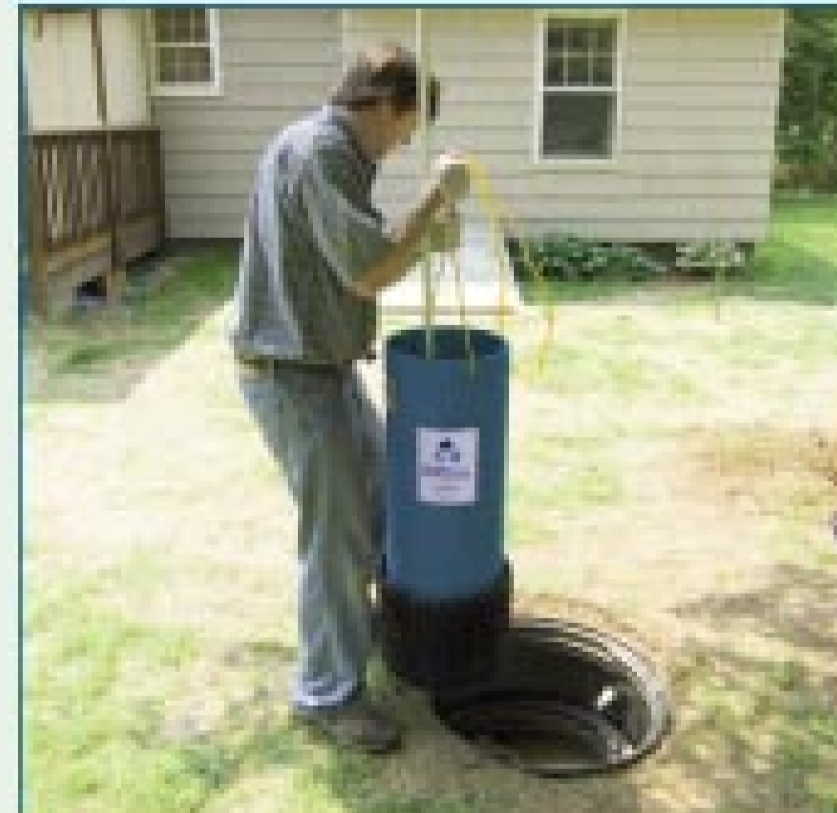
Aquaworx Remediator Installation
