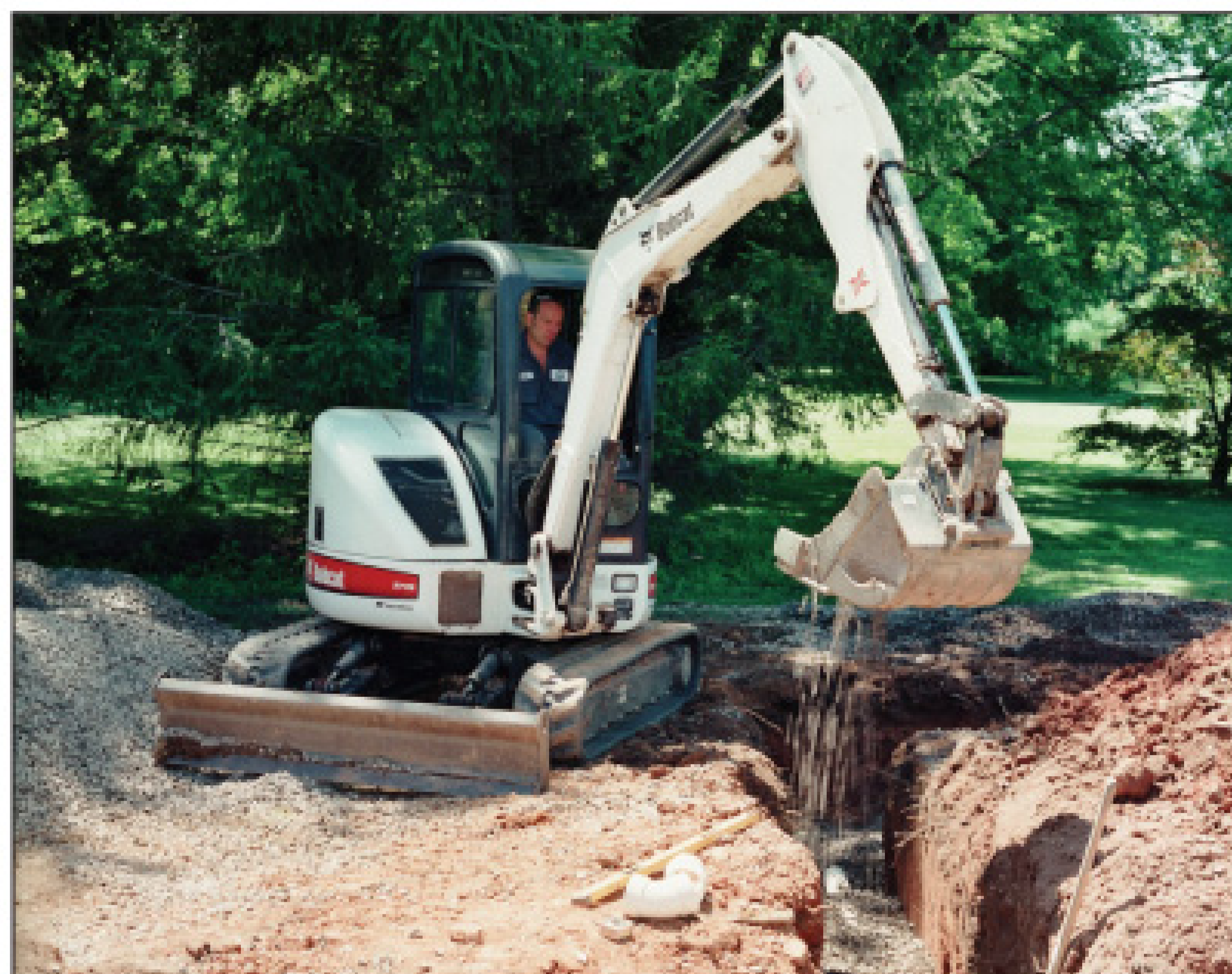
Michael Biros backfills stone bedding for a septic system delivery line.
