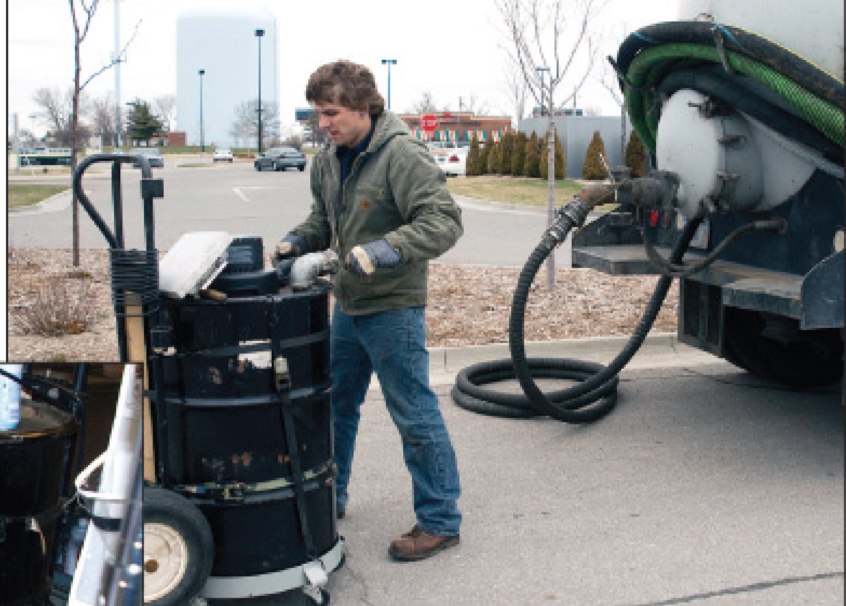
Grant Horton uses a Wee Vac from Wee Engineer Inc. to clean a grease trap. The portable vacuum is used for traps that can't be accessed by a truck.
