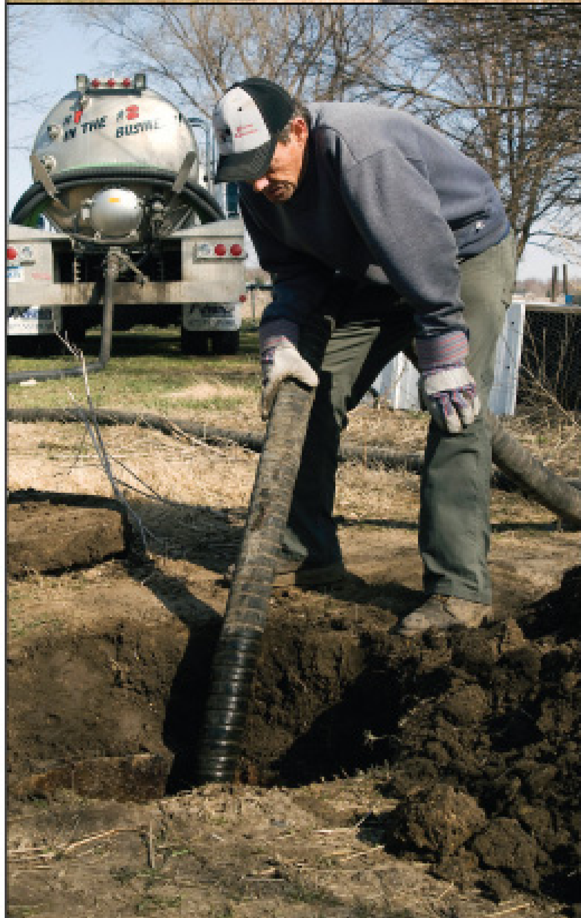
Mike Ribordy (left) pumps a septic tank, while a septic system (above) is exposed for a time-of-sale inspection.
