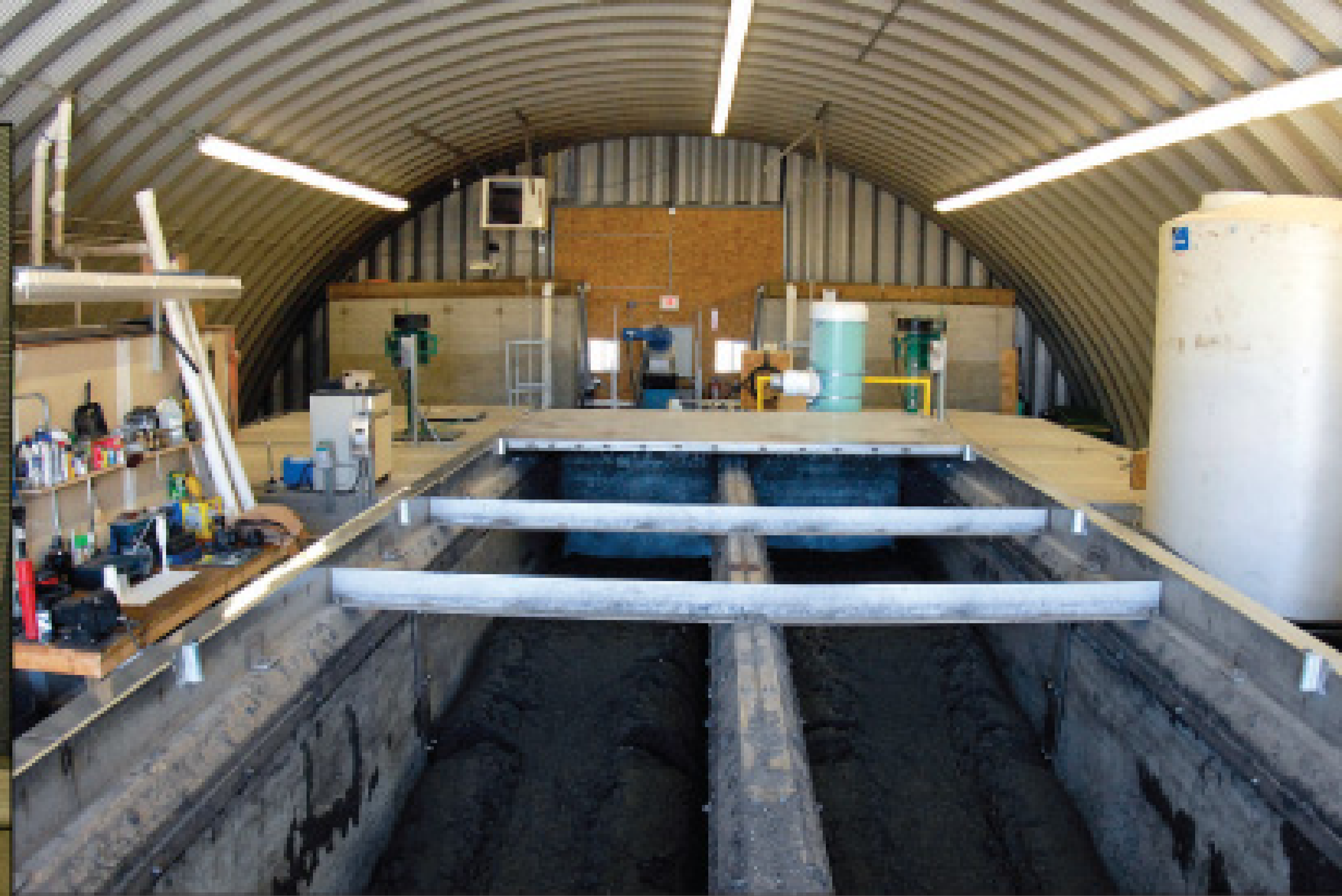
Jerry Heckman, plant superintendent, adjusts the sludge agitator (left) and adds polymer to the waste that's treated in the 50- by 70-foot facility.
