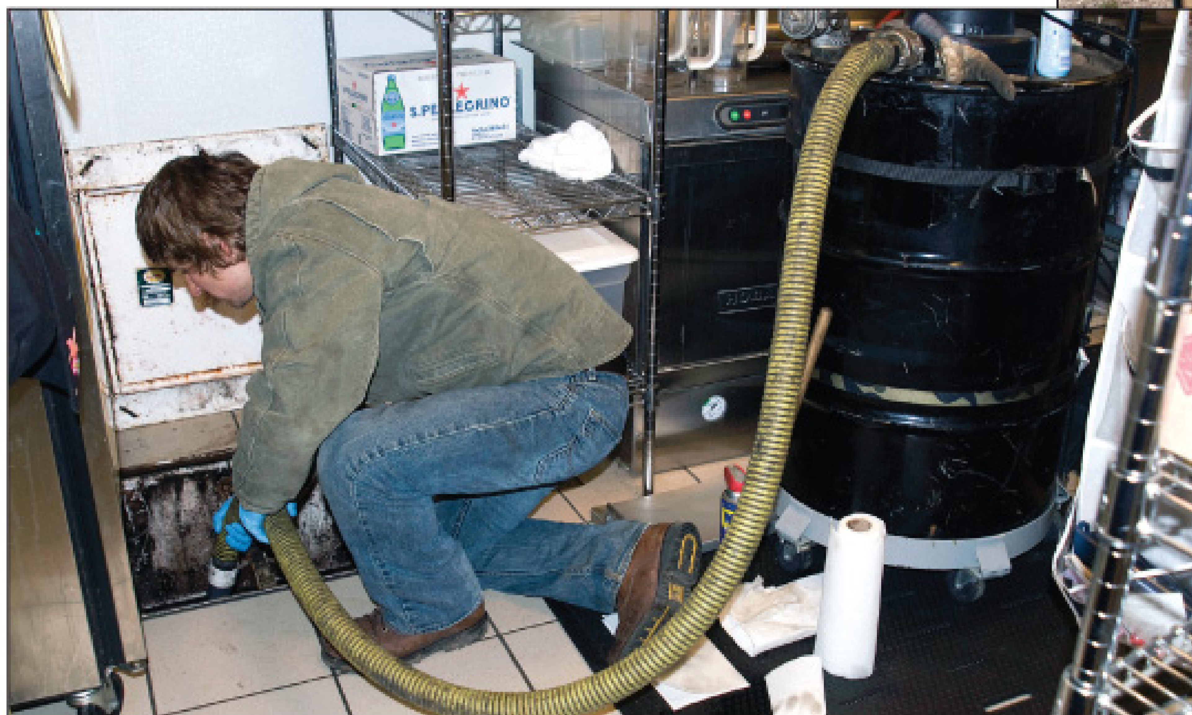
Grant Horton uses a Wee Vac from Wee Engineer Inc. to clean a grease trap. The portable vacuum is used for traps that can't be accessed by a truck.
