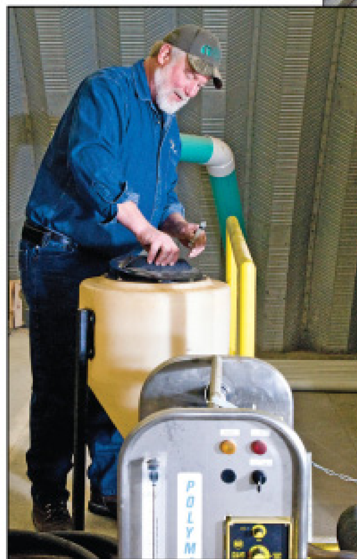
Jerry Heckman, plant superintendent, adjusts the sludge agitator (left) and adds polymer to the waste that's treated in the 50- by 70-foot facility.
