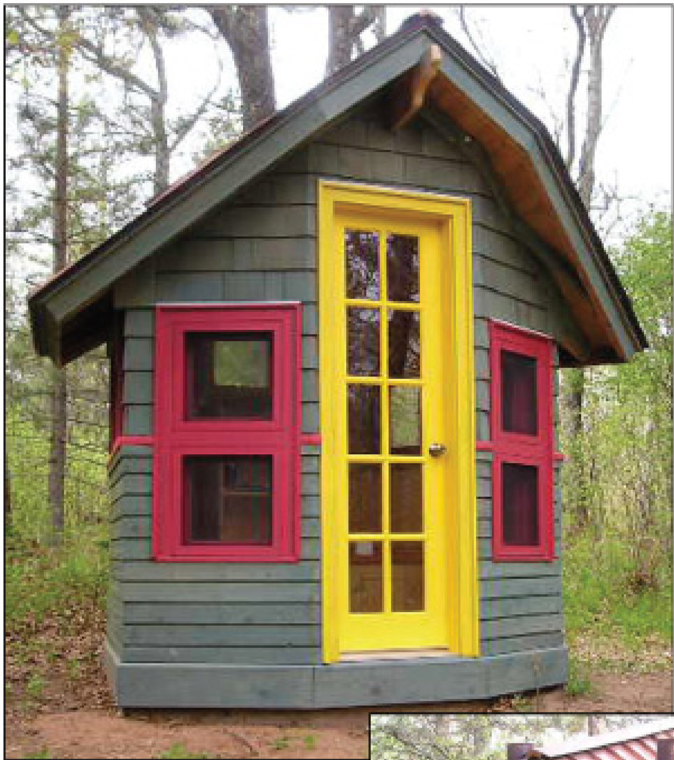
At left: A welcoming entrance greets the guys who walk through the woods to get to Sylvestre's outhouse. Below: The sloping copper roof helps make the outhouse an out-of-the-ordinary architectural gem.
