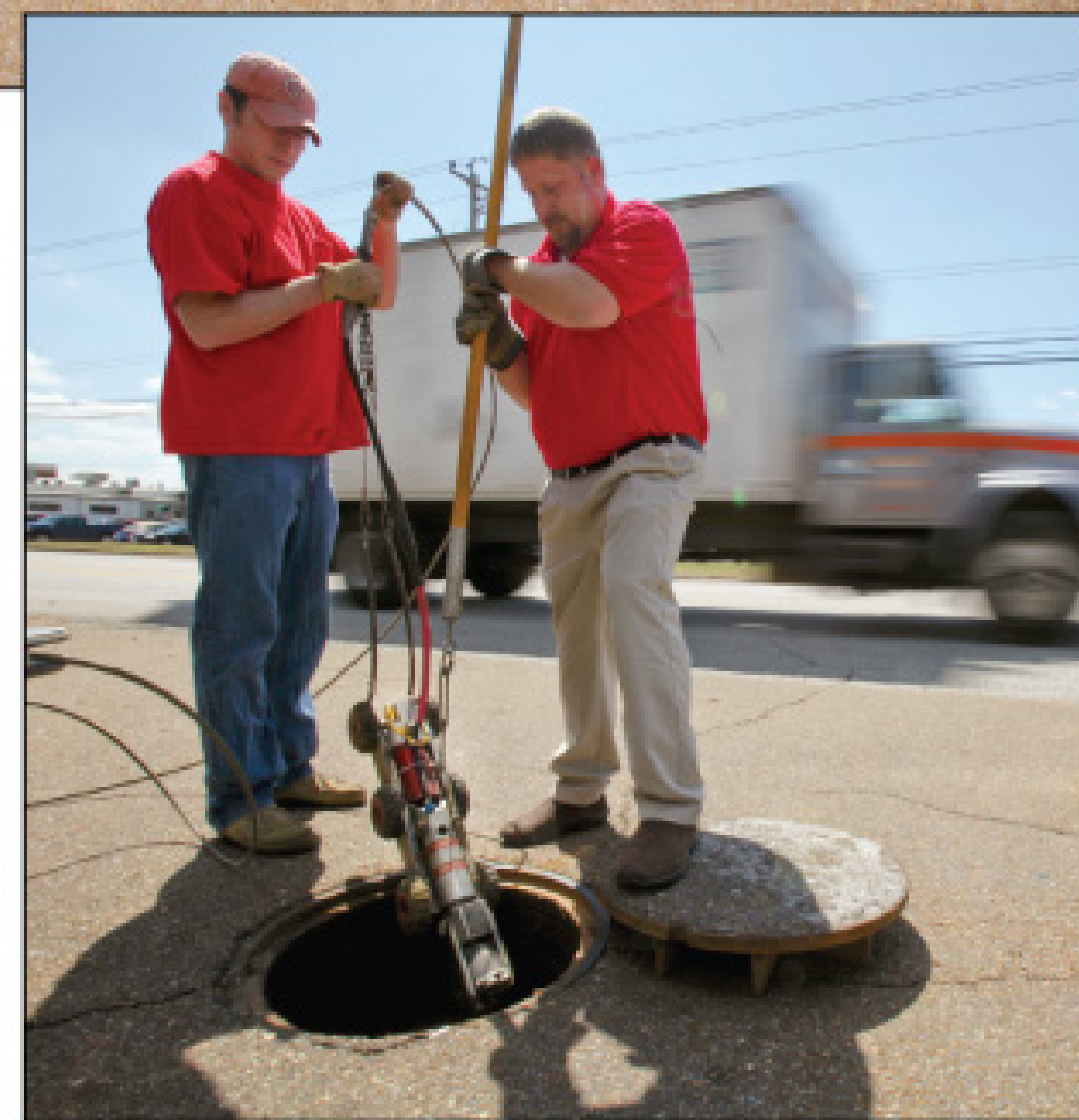
Lucio Puente cuts an entry hole for a water line repair under a car dealership parking lot.
