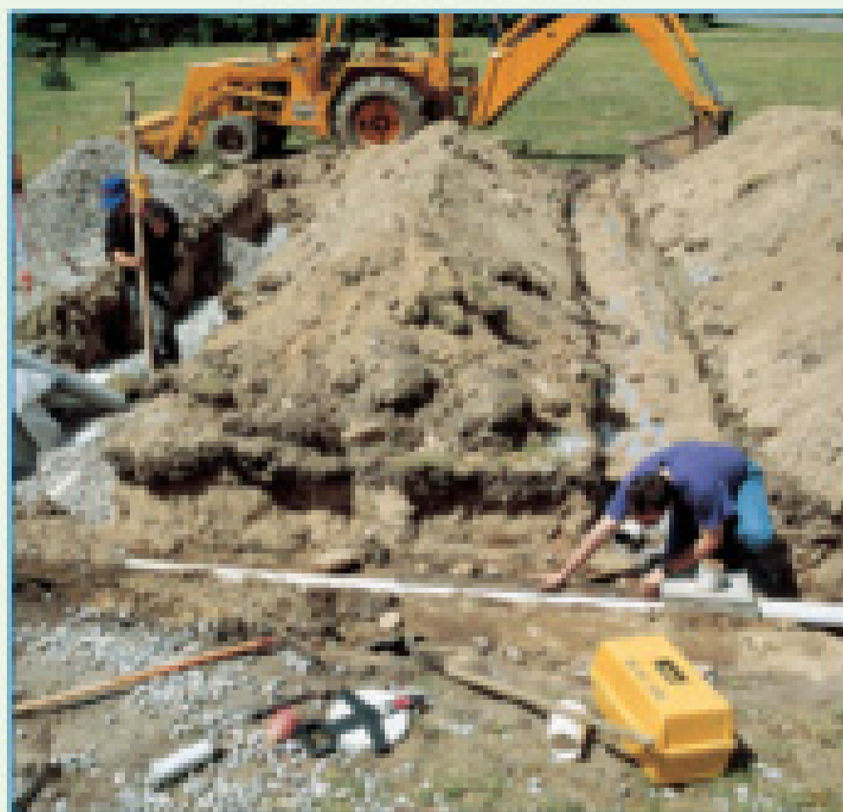
Typical Septic System Replacement Installation
