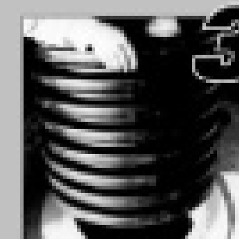
Place plastic riser pipe over ring.
