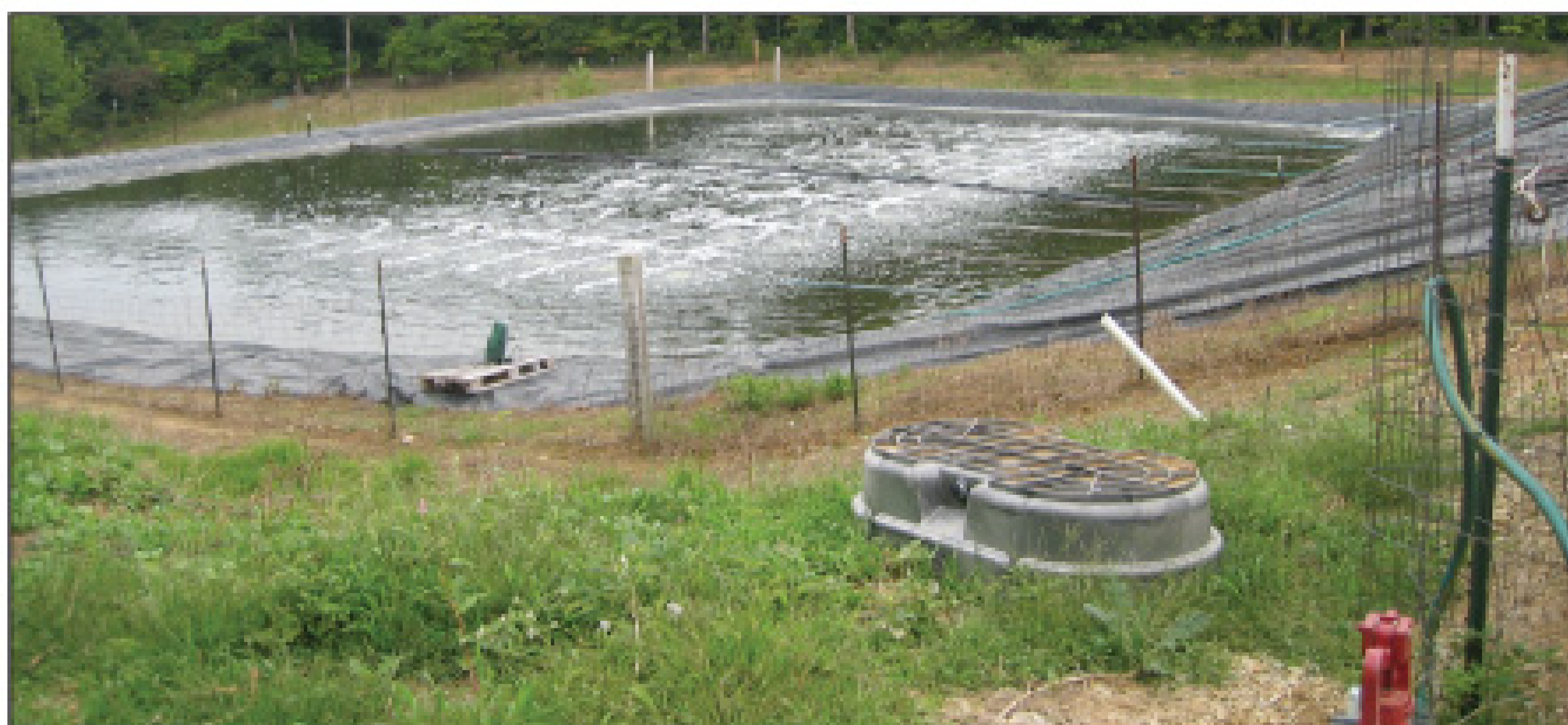
Above: After treatment in one of four effluent lagoons, waste is chlorinated and discharged to a stream. At right: Symposium attendees inspect the automated Lakeside Septage Acceptance Plant.
