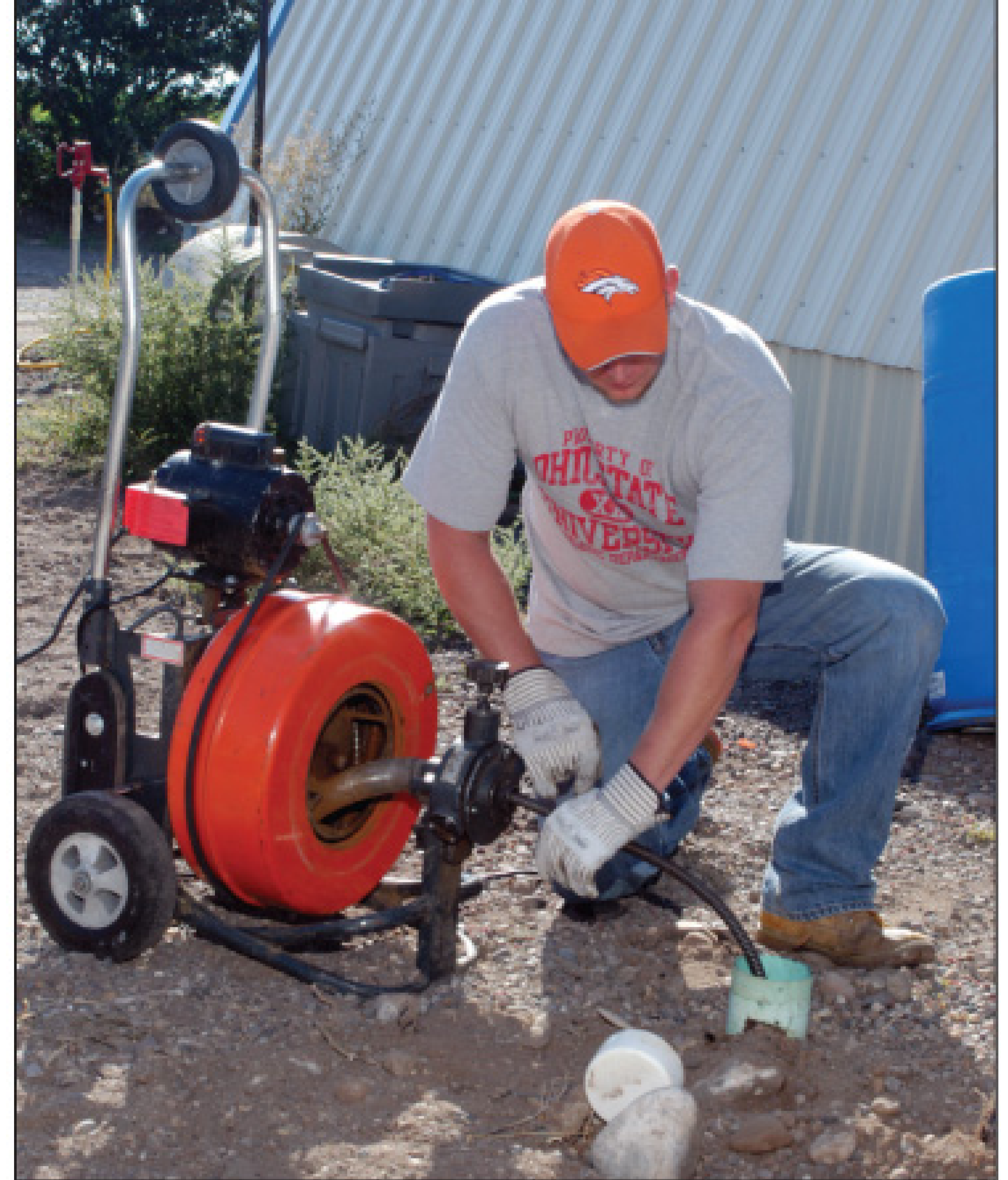
Leonard Brown pumps out a septic tank before he and his son, Russell, dig it up. At right, Russell cleans a sewer line.
