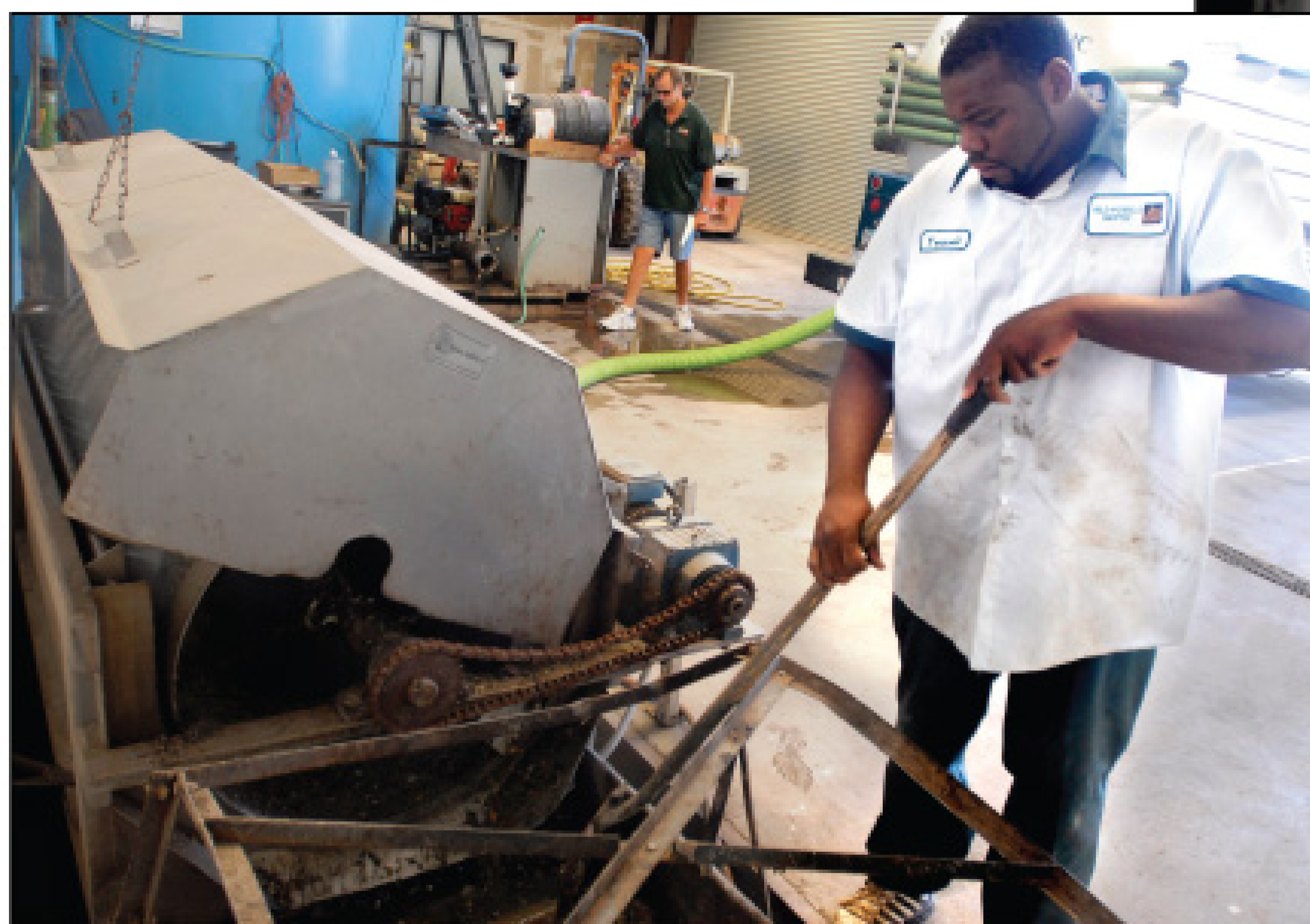
Above, septic technician Terrell Hill (left) and Steve Ziegler drain waste from a pump truck prior to processing. At left, Hill cleans debris and trash filtered from the sewage strainer.
