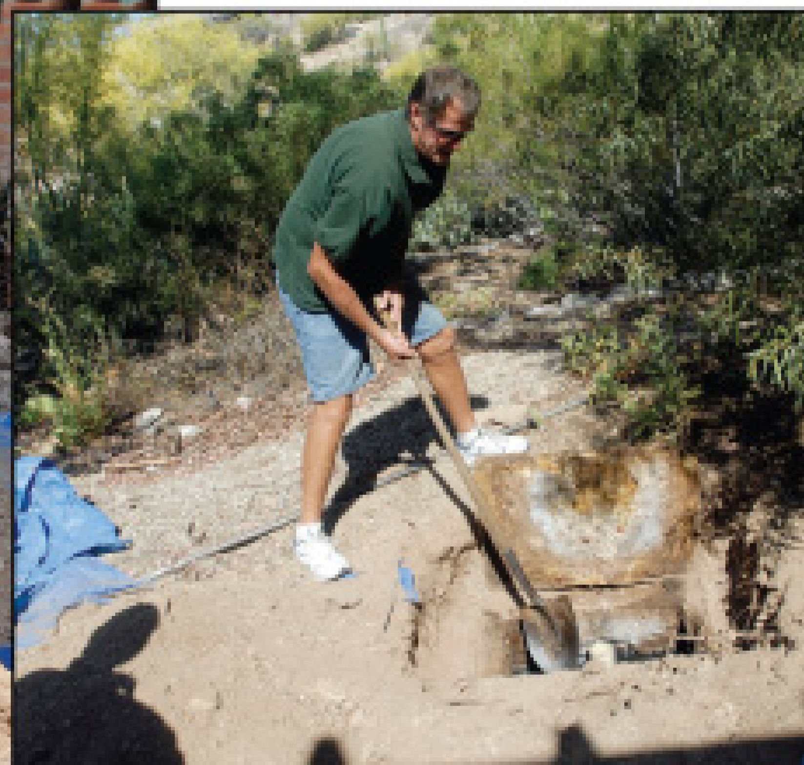
Steve Ziegler helps Zep Holmes open a septic tank, then checks to see if another lid needs to be removed.
