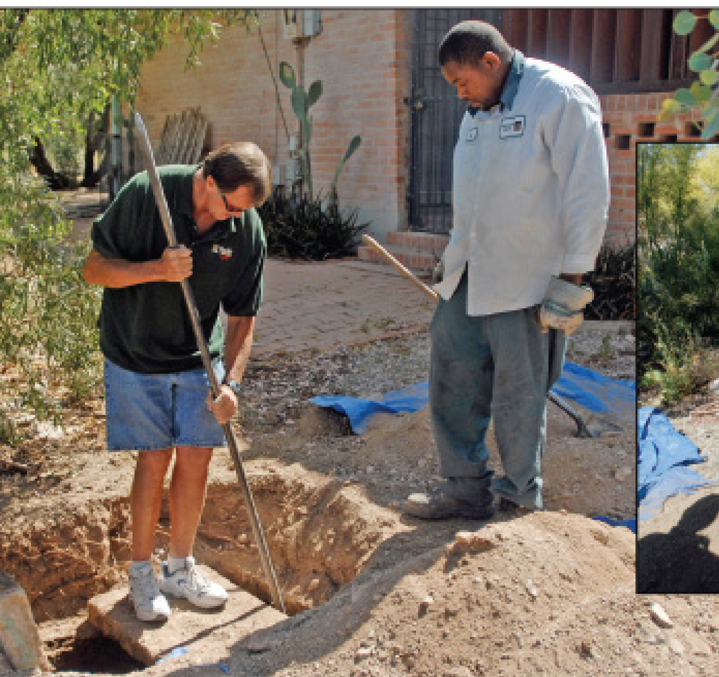
Steve Ziegler helps Zep Holmes open a septic tank, then checks to see if another lid needs to be removed.
