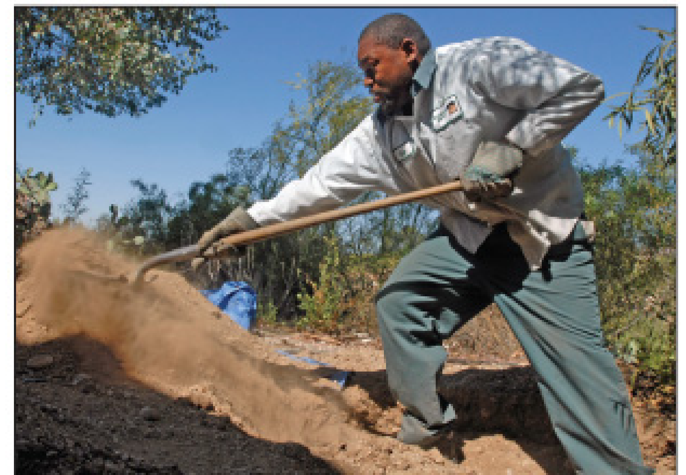
Steve Ziegler helps Zep Holmes open a septic tank, then checks to see if another lid needs to be removed.
