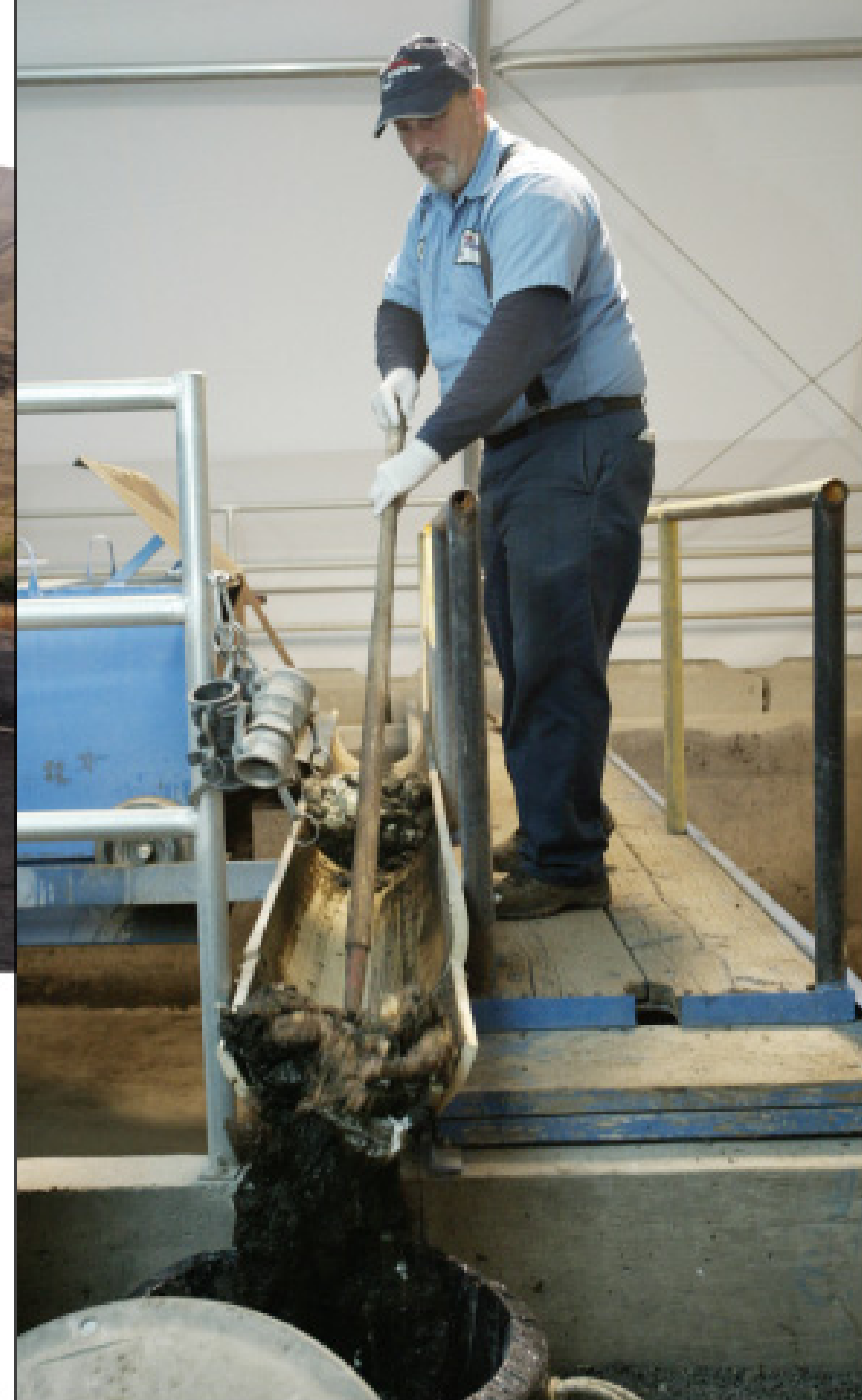
Scott Meyer, a partner in Clearwater Tech, moves large debris filtered from a load of wastewater in the first step in the company's dewatering process.
