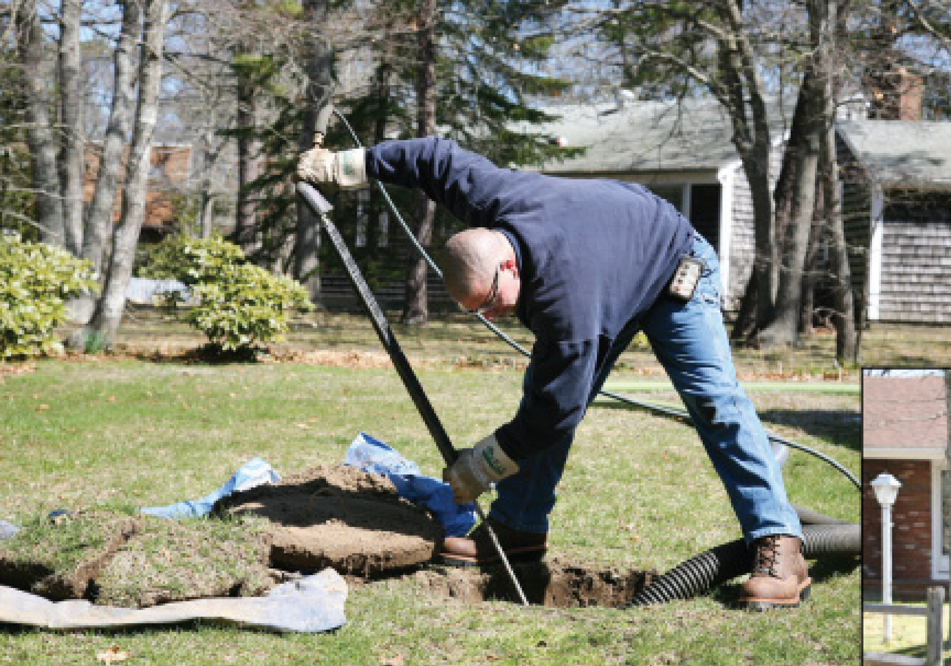
Above, technician Paul Martin jets a septic system at a residence in Hyannis, Mass. At right, Martin hooks up a hose to the Juggler truck before pumping a septic system.
