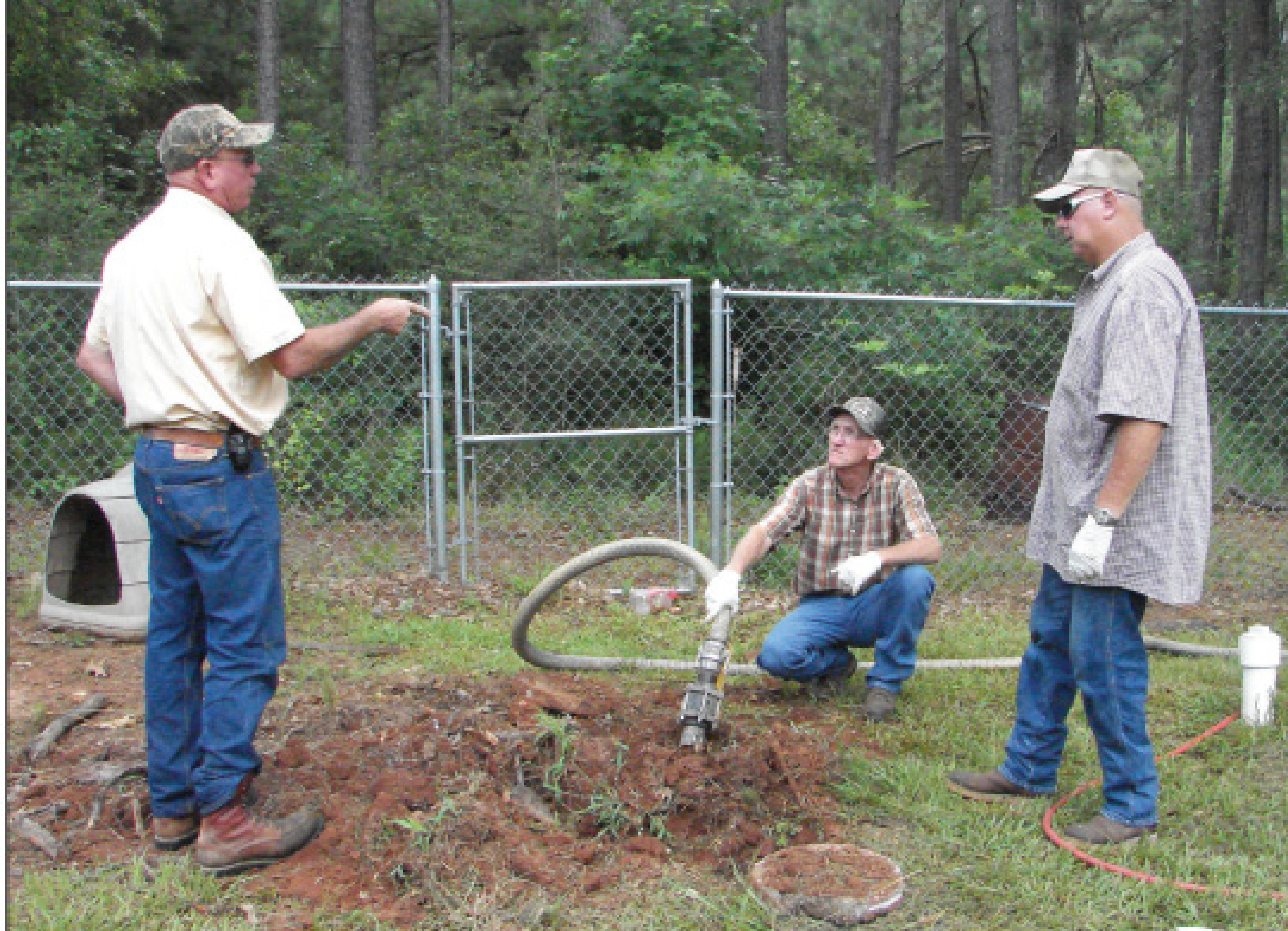
Jeff Martindale (left) checks with technicians Mike Dickerson and Thomas Ward as they pump a residential septic system. Martindale is often on the road, and flies his own plane to save travel time between appointments.
